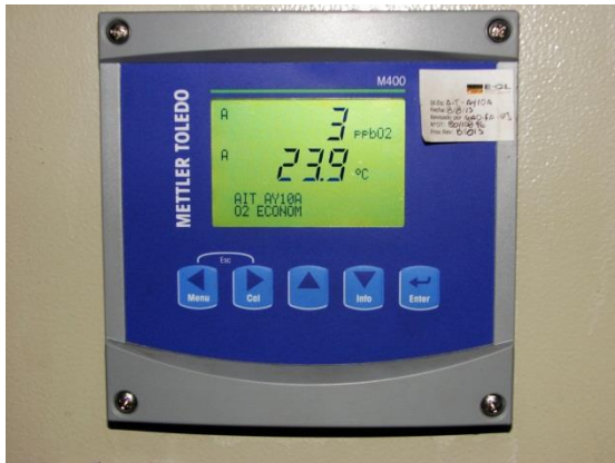
Oxygen Sensor in economizer.
